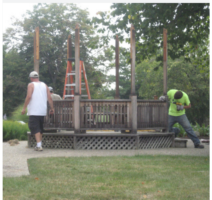
Workers dismantled the old gazebo on July 29.
