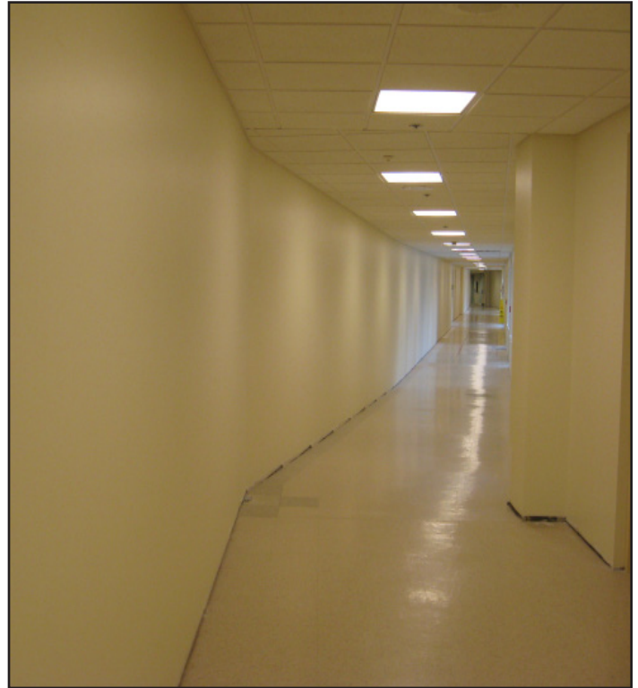
The waterproof walls are now installed in the "tunnel" (Building 6, Level 1)
