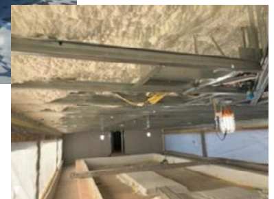
View from the rafters with spray foam insulation applied
