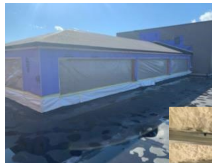
The exterior as seen from the roof
